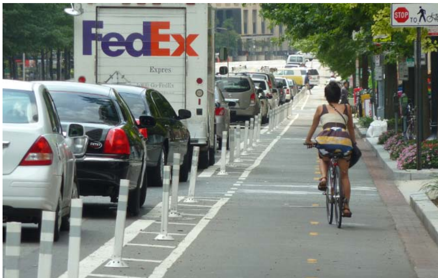
The 15 th Street Cycletrack in Washington, D.C. (above) is similar to the planned cycletrack for Baltimore where Parked vehicles (left) and a striped buffer (center) provide cyclists 2 layers of separation from moving traffic.
